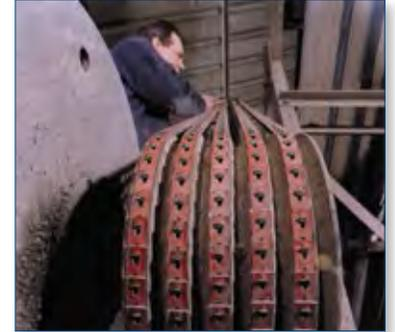
**Solution** *Installing NuTLink V-Belts reduced downtime to just two hours with the added bonus of longer belt life.*
